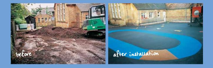
Wet pour base specification (variable thickness 30mm & over)
